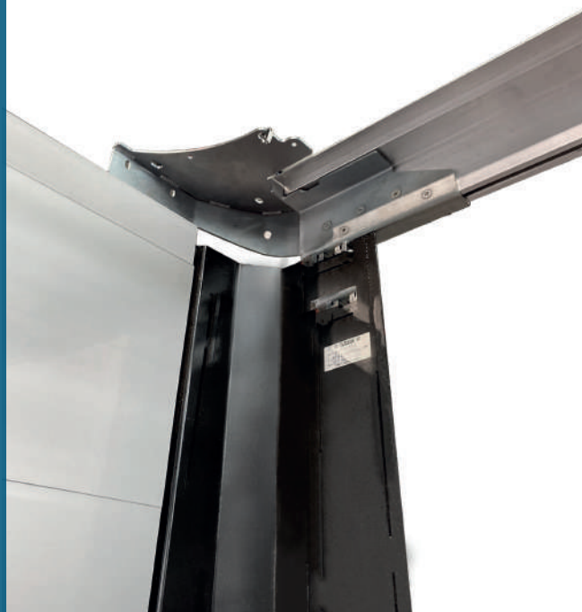
Vista interna Detail from inside
